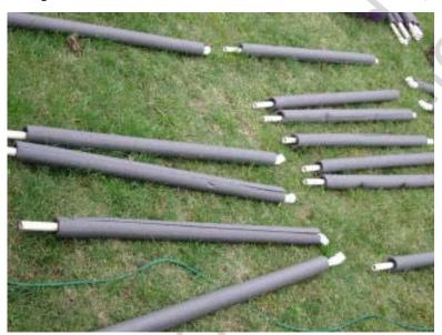
The leg pieces are sorted out. Each one is marked with the leg (letter) and joint (number).
