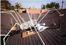
Each spider leg is constructed in layers. This photo shows one leg for each layer: inner skeleton of PVC pipe, meaty layer of foam pipe insulation, and fabric skin.
