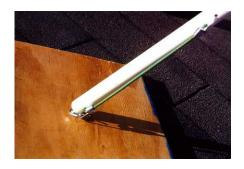
Six of the spider's feet touch the roof. Those legs don't need to be terribly strong, because they are supported at both ends. This is a foot pad, which anchors the far end of the legs.
