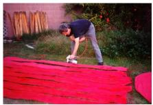
Everything that touches the roof has a plywood base, with carpet scraps facing the roof. This is the main base for the spider body. It is upside-down, with carpet scraps being applied with <a href="https://hot-melt.glue">hot-melt.glue</a>.
