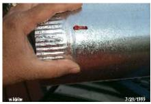
Here you can see how the ties connect to the stove pipe. I drilled two small holes for each tie and then just looped the tie through one loop of the coil and through the holes. Start by leaving the loop loose, and attach the coil at three points around the stove pipe, then tighten the loops a bit at a time till the
