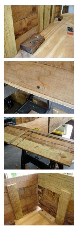
Pre-drill and screw in 1 3/4 " screws in three places on the wood anchor. Use two wood anchors for the one side. Repeat process to attach the other side to the bottom.
