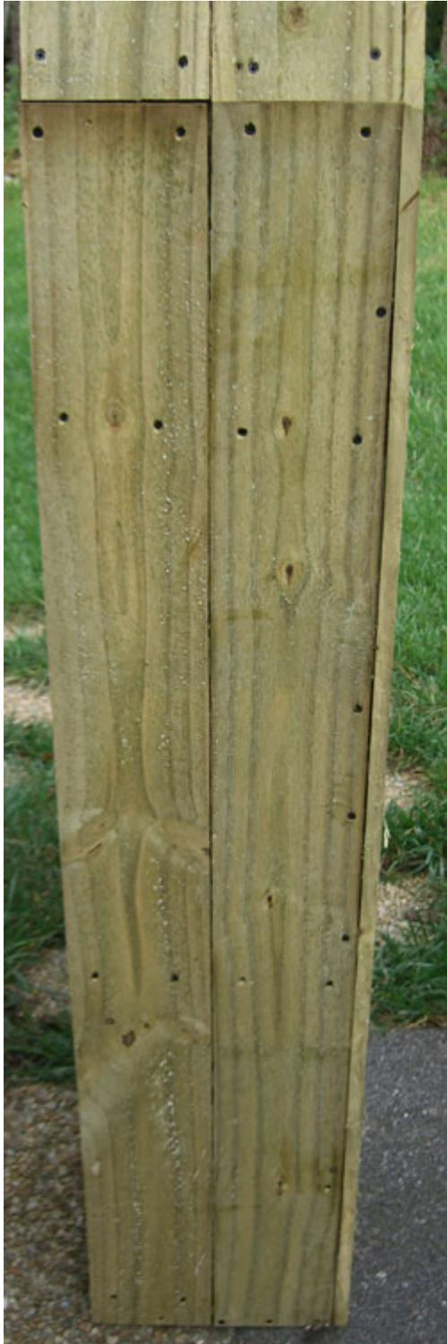
The lower sidewalls were also screwed to the vertical ribs and the sidewall support pieces attached to the bottom.
