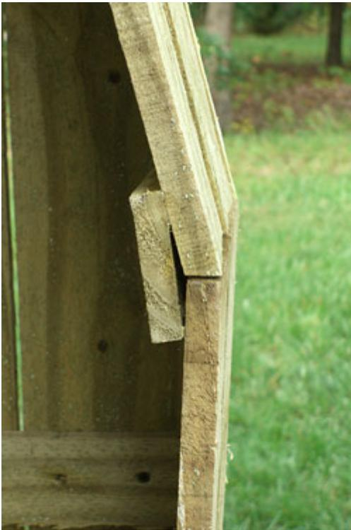
One of the vertical ribs was used to secure the angle at the shoulder area of the coffin. This was probably the weakest joint so extra glue and screws were used.
