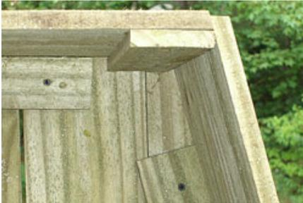
The vertical ribs also provided the support and gluing surface for the corners of the coffin.
