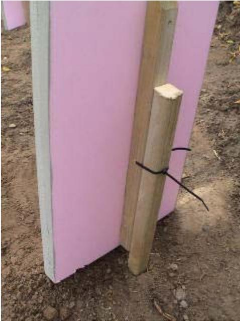
Here you can see the "zip-tie" going through the hole and around the stake. It is VERY secure as the bottom of the stone keeps it from tipping to the side and the friction of the wood on the wood keeps it stable.
