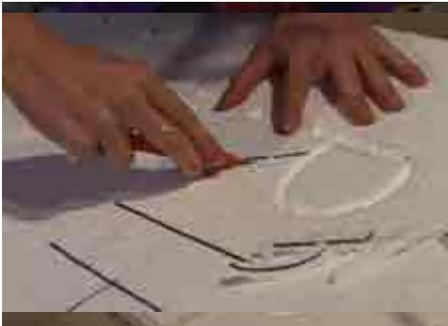
The best way to get 'em to stick is to apply a little glue and then (and most importantly) take some small nails or even straightened-out paper clips (anything small and rigid) and stick it through the small piece tacking it onto the big piece. You're essentially "nailing" the brick to the headstone.
