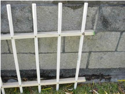
I slid the PVC through the holes and screwed each pipe in place with a single sheetrock screw.
