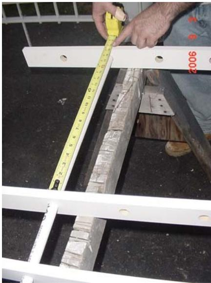
Christopher switched to weather resistant wood and pre-drilled and countersunk holes for all the screws, making for a much neater and more sturdy fence section.
