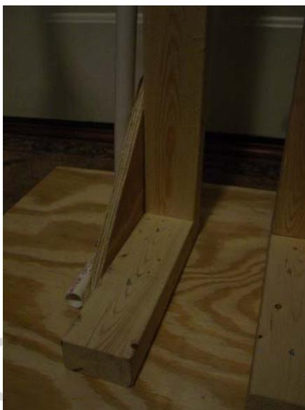
Shot of the "L" supports I added. They are simply 2"x3" screwed together with a plywood triangle added for rigidity.
