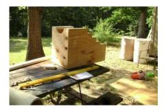
I took my time and nailed it together, also used screws for strengthening the frame. The front panel I cut out a half circle at the top so the pvc barrel would lay into the frame.
