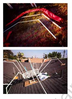
Each spider leg is constructed in layers. This photo shows one leg for each layer: inner skeleton of PVC pipe, meaty layer of foam pipe insulation, and fabric skin.
