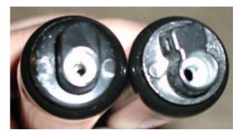
The hole for the valve screw is in two parts. The outer part is wide enough for the head of the screw to go in. The inner part is narrow, and threaded to accept the screw.
