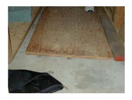
2. Now, nail the thin length wood in place from the top of the plywood boards. That is, the pointy sides of the nails should be in the thin length of wood, and the heads should be flat with plywood board. You may need to use other wood to prop up the board's sides so that it doesn't wobble while you're nailing.
