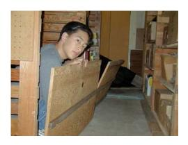
The floor is made of two boards of plywood supported down the center by a thin length of wood. The first board is stabilized with additional supports underneath, but the second board rocks freely from side to side, only supported in the center.
