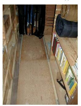
4. Once you have your wooden floor built, you will need to add something to prevent people from tripping when they step onto the board. I laid a long piece of carpeting across the entire floor and taped the ends down with duct tape. This created enough of a ramp that guests would not trip, while still allowing the board to rock. If you are so inclined, you could build a wooden ramp up to the raised board, or sink the board into the ground if the situation allows.
