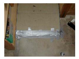
5. If you have any space to either side of floor, use other pieces of wood to make it level with the raised walkway. You don't want someone's foot to get stuck between the wall and the floor.
