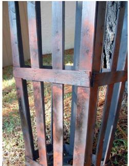
It is up to you how you put all the sides together to form the finished cage. You can purchase L shaped brackets, you can cut and put small pieces of wood in the corners and screw each side into them or you can simply drill holes at various points in the front and side and run thin gauge wire between to hold it together.
