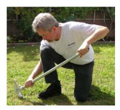
Dennis uses a conduit bender to form the upper piece of rebar into the 90-degree bend.
