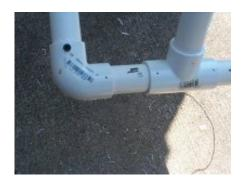
Here you can see that a small hole is drilled into the PVC connector and a decking screw screwed into the hole. This is how I secured the frame. Cement could be used but the frame tends to take a lot of abuse and the cement did not seem to hold up as well.
