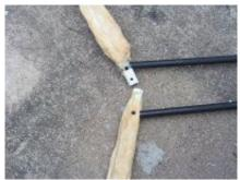
The rods are connected to the arms by drilling a hole in the arms the same size as the rods and then using a deck screw to secure them.
