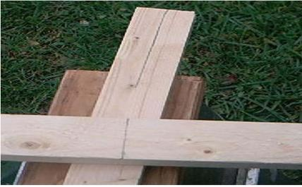
I started off by marking the center of the furring strips with a pencil so I could join them together square and true. I found the center of the shorter furring strip by dividing its length in half. The center of the longer strip is half the width of the furring strip itself. When you line up the pencil marks and square the two pieces at the top of the "T", you have a nice, regular "T" shape.
