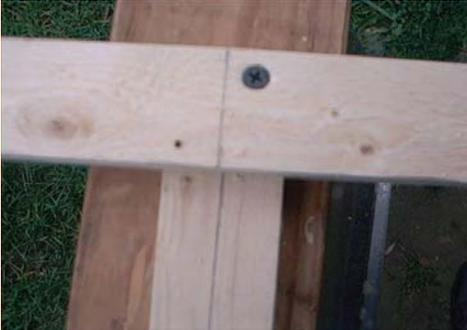
I fastened the furring strips together with 4 1" drywall screws. I predrilled the holes with a small drill bit and an electric drill. You want to predrill the holes to keep from splitting the soft wood. You can see one of the predrilled holes left and below the drywall screw on top. I then flipped the "T" over and put two more screws in the opposite corners on the other side. The drywall screws do a good job of making a tight joint. A little bit of wood glue would even make the joint stronger.
