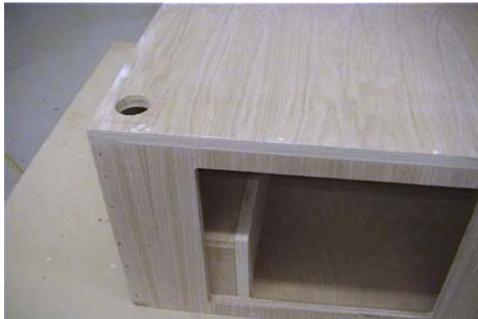
Access inside this box will be important while installing the mechanisms that will run our prop. Here is a look at the underneath side of the floor. You can see that I have used face frame screws and pocket-bored to the sides and front so that I would have the strength of screws without the head of the screw showing. This turned out to be a non event, as I had many screw heads exposed by the end of this construction anyway and they weren't even visually evident.
