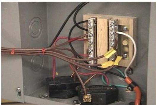
Looking inside the box you will see a piece of plywood was used to mount some 110V gang connectors to that will serve to make this steel box a power panel for the chair.
