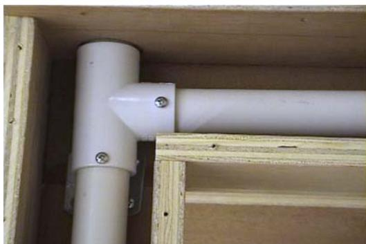
As you can see, the drain pipe winds up just recessed from the bottom of the floor where the side of the pedestal will be attached. Don't forget your access opening to the drain plug! 3" square opening should suffice.
