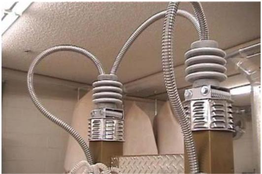
To the two bolts on top of the insulators I screwed some flex conduit connectors that I had ground down on angles so they would send off my decorative conduit in different directions, so that it looked authentic when attached.
