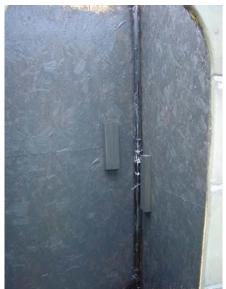
In 2006, I rebuilt the crypt's frame to include 1/2" OSB to strengthen it and keep it all from getting blown over like it did last year when it was all PVC and foam. I also built it to be taken apart easier and cut all the large pieces of foam and OSB in half so it can be stored easier. I used 14 gauge wire to hold the OSB to the PVC frame, and then used scrap pieces of 2"X4" to brace the OSB together.
