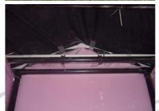
All of the roof structure is made from 1" PVC since I had a lot of that laying around. After I got the frame for it built, I covered the top of it with some black plastic to help keep any moisture from leaking through and used duct tape to attach it to the PVC. Then I cut
