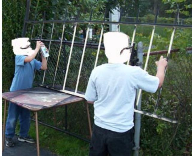
**Once done, you're ready to display your fence. Find some rebar, or metal rod or threaded rod. Pound into the ground and slide each end of the fence over it, into the pvc (you might want to remove the screw in the piece of pvc first).**
