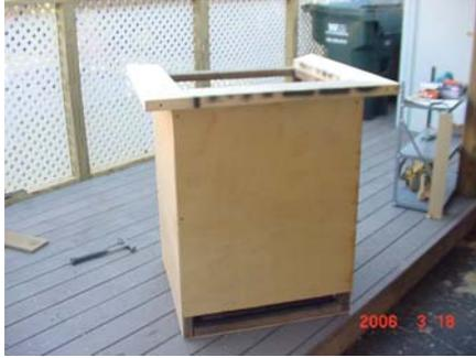
Last step in the carpentry phase was to build a lip/sill around the top of the well. We've left the back of the well open for the time being since we'll need to be inside there a bit mounting the electronics and pneumatics.
