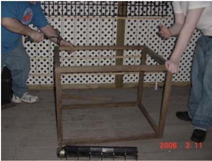
First, fabricating the box/frame from 2x2s. 3 feet tall, 27" wide on each side (a 24" 2x2 with outer 2x2s nailed to it).
