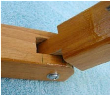
The legs consist of wooden 2x2's (approximate dimensions below). The leg joints are just simple tongue and groove cuts joined by a #10 screws, washers and nuts.
